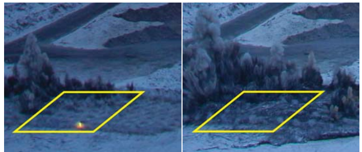
The 48 holes using Rocklock stemming plugs (highlighted) show an increase in gas energy containment.
